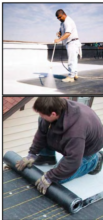
Figure 6: Two Cool Roof Installations
